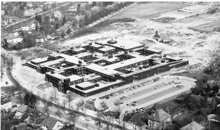
3 - Approximately one quarter of the competition project was built.
