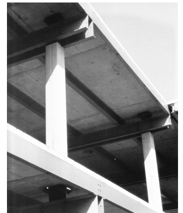
5 - A simple, prefabricated structure.
