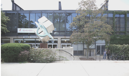
Entrance to the Galvin Library at the Illinois Institute of Technology. Built by Skidmore, Owings & Merrill
